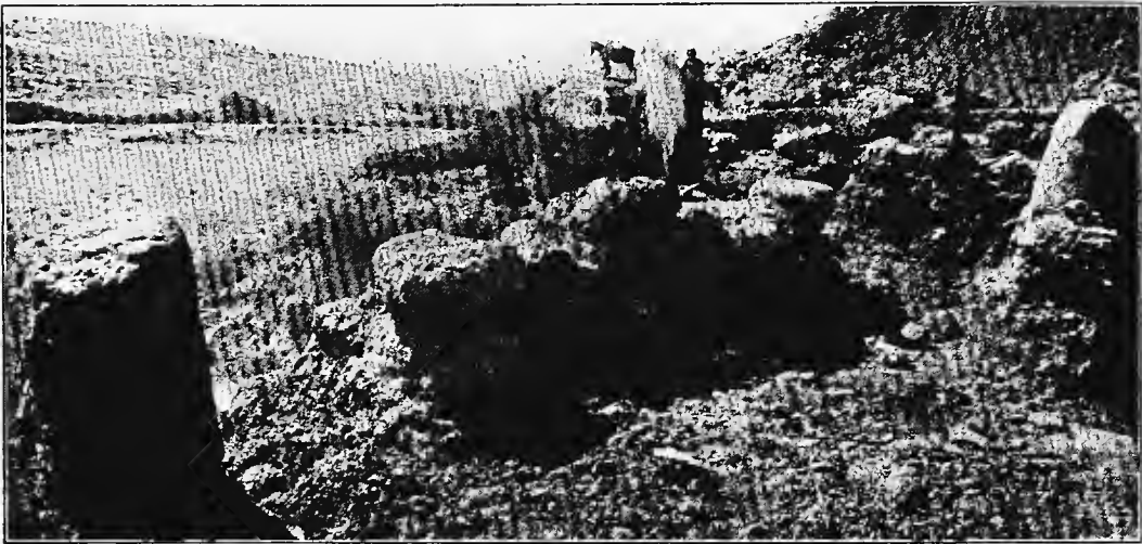
FIG. 65.—WALL CONSISTING OF A ROW OF LARGE STONES WITH SMALLER STONES BETWEEN THEM
